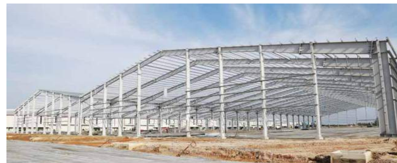
Pre-engineered building construction
