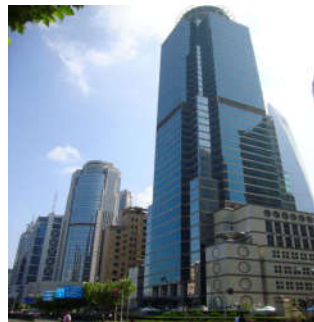
SHANG HAI New Shanghai International Tower, Shanghai, China
