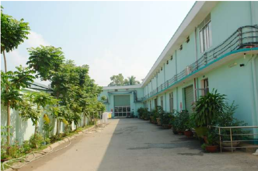
The Factory Internal Road
