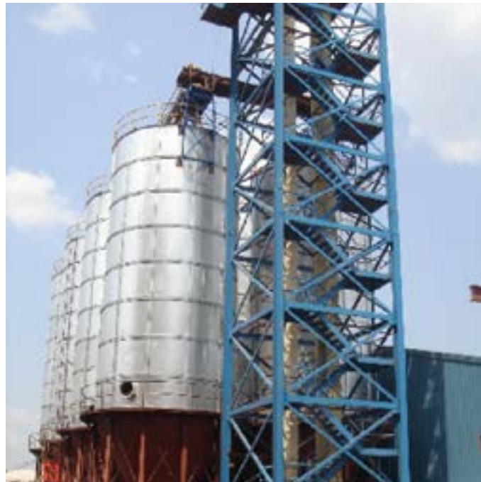
Bucket system and material storage cylinder
